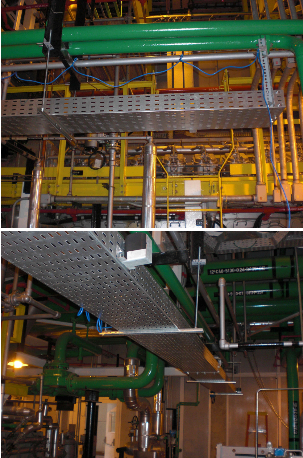
Figure 5.3: The industrial plant where the videos of the VDAO database were recorded.
